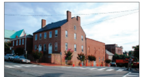
Fredericksburg No. 4 with chimneys before removal
